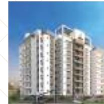
DEEPAM 2,3&4 BHK APARTMENTS VATTIYOORKAVU, TRIVANDRUM
